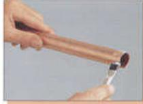
**1.** These combinations of materials require the use of a non-aggressive, water soluble flux. Using a brush or a clean rag apply a small amount of flux to the end of the tube and to the inside surface of the fitting. Avoid overloading and spilling flux inside the tube itself as the residue **needs** to be removed on completion of the joint.
