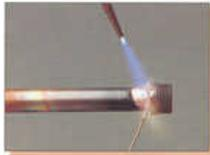
**2.** The procedures for these joints are essentially the same as for Copper to Copper jointing, only that more heat should initially be concentrated on the brass or copper-alloy fitting to bring it to temperature. Take care not to overheat the fitting. Dull red colour is sufficient.
