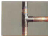
**5.** To complete the joint, an even build-up of solder should be **just** visible around the shoulder of the fitting. Remove the heat (taking care not to disturb the joint) until the molten brazing alloy solidifies to a tan black colour (approx. 10-15 seconds) After brazing is completed, the joints are normally left to cool in the air. However, if necessary the joints may be quenched in water or cooled with a wet rag.
