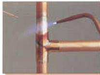
**3.** Apply heat uniformly to both tube and fitting, by moving the torch around to ensure even heating before adding the silver solder.
