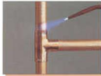
**2.** Push the tube tightly into the fitting or the expanded end of the other tube and apply heat. Brazing torches fuelled with air-acetylene, propane-oxygen or oxyacetylene torches are all suitable.
