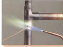
**6.** To braze an upwards vertical joint follow the same procedures, although more heat should be concentrated on the fitting than the tube. This will draw the molten brazing alloy upwards into the capillary gap.
