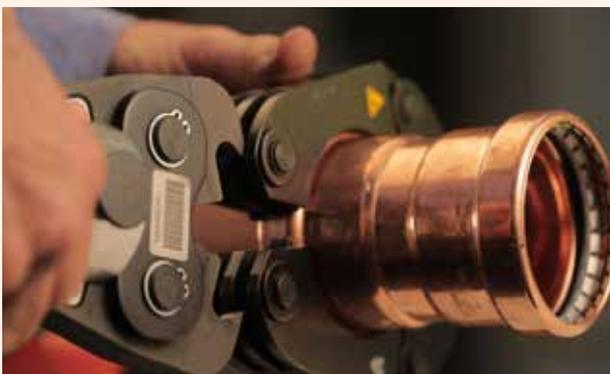
**9.** Open the ZB203 Adaptor Jaw by depressing the jaw levers and attach to the press collar so that the claws of the jaw grip around the pins of the press collar. Initiate the pressing job by pressing the start button. The pressing procedure should not be interrupted prematurely unless in an emergency by pressing the emergency stop button. The KemPress tool will flash if the fitting does not press correctly.
