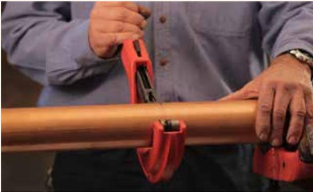
**1.** Cut copper tube to length using a pipe cutter or fine tooth saw and ensure the pipe is cut square.
