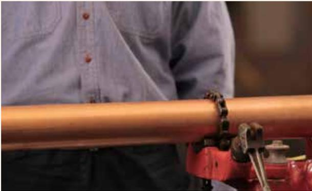
**5.** Secure the tube in a vise or pipe support to prevent any movement of the tube and insert the fitting onto the tube. Ensure the outer edge of the fitting lines up with the insertion depth mark made in step 4.
