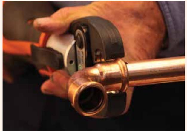
**7.** Check the fitting outer edge still lines up with the marking. Open the pressing jaw and close it around the fitting so the raised bump in the fitting rests inside the groove of the pressing jaw. Ensure the jaw is engaged square with the fitting and not on an angle.
