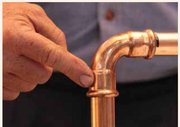
**9.** Visually inspect the fitting to ensure the press has been completed. The KemPress® tool will flash if the fitting did not press correctly. If this occurs a new fitting and tube section is required. At the end of the project visually inspect each fitting to ensure none have been missed.
