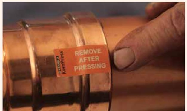
**10.** Release the adaptor jaw from the collar and the collar from the fitting. Remove the KemPress® label to indicate completion of the press.
