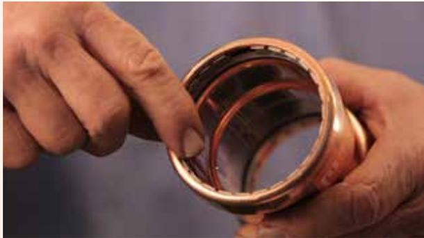
**3.** Ensure you have the correct sized fitting, check the fitting is clean and the stainless steel grip ring and O-ring are free from debris and correctly seated in the fitting.
