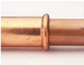
Unpressed fitting - smooth with no indents.
