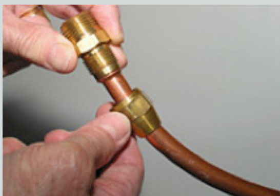
Figure 7.1a Assembling Copper Flare Pipe Adaptor and Nut
