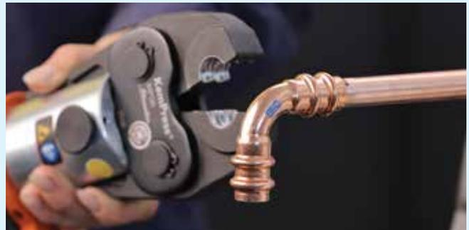
**10.** Attach the jaws onto your KemPress KPL3 tool or other compatible full size 32 Kilo Newton press tool and lock it by engaging the locking pin. If using a KemPress KPS2 press tool, ensure you use Streamline ACR Press small jaws, as large and small tool jaws are not interchangeable.
