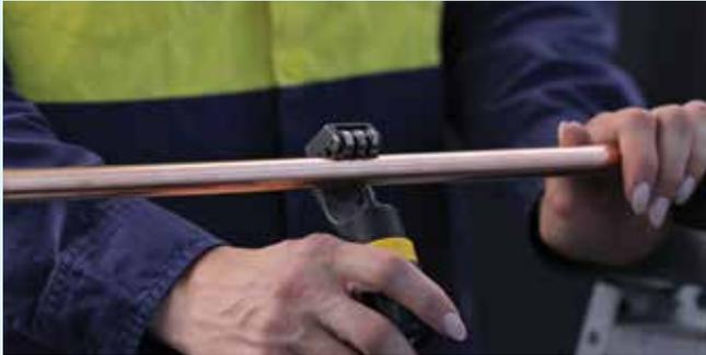
**1.** Select your AS 1571 copper refrigeration tube. Using a tube cutter, cut the tube to the length required ensuring the tube is cut square.
