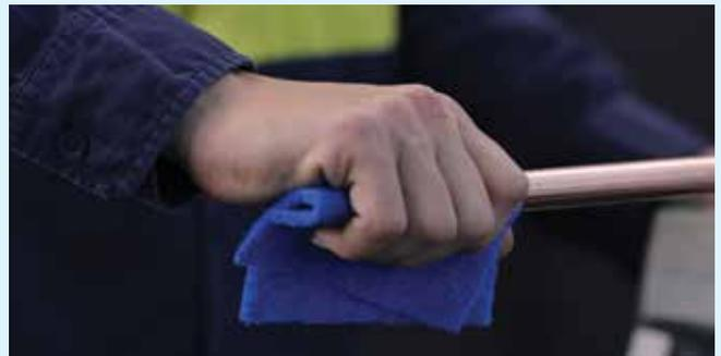
**4.** Clean and smooth the tube surface using an abrasive pad, emery paper or a soft medium grade scourer. Ensure the tube surface is free of indentation, scratches, deformation, oxidation and dirt or debris.
