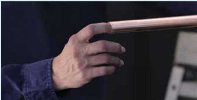
**3.** Ensure the tube ends are free of any burrs or sharp edges that might damage the internal components of the fitting.
