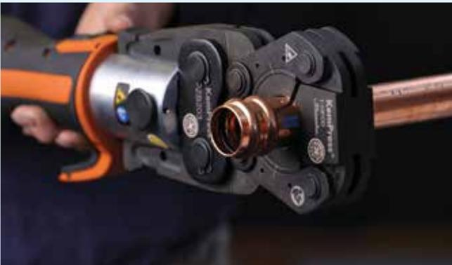
**15.** Check the fitting is still fully engaged to the insertion depth mark and once the jaw and fitting is correctly engaged, initiate the pressing process by holding down the start button.
