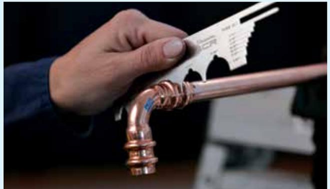
**16.** Verify the connection is secure and complete by using the Streamline ACR press gauge between the pressed O-ring beads. Rotate the gauge to avoid interference with flashing. If the gauge for the corresponding fitting size fits, the press has been completed.
