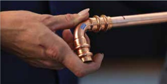
**7.** Insert the fitting, slightly rotating the fitting whilst sliding it onto the copper tube.
