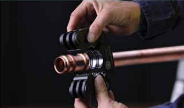
**13.** Open the press collar and place it over both beads of the fitting at a right angle to the copper tube. Ensure the two beads of the fitting fit into the two corresponding grooves of the press collar.
