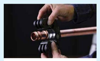
**13.** Open the press collar and place it over both beads of the fitting at a right angle to the copper tube. Ensure the two beads of the fitting fit into the two corresponding grooves of the press collar.
