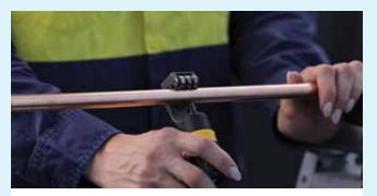
**1.** Select your AS 1571 copper refrigeration tube. Using a tube cutter, cut the tube to the length required ensuring the tube is cut square.
