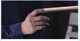
**3.** Ensure the tube ends are free of any burrs or sharp edges that might damage the internal components of the fitting.
