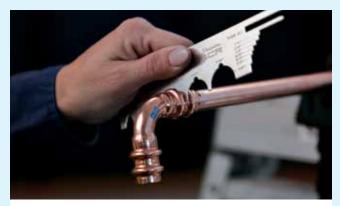
**16.** Verify the connection is secure and complete by using the Streamline ACR press gauge between the pressed O-ring beads. Rotate the gauge to avoid interference with flashing. If the gauge for the corresponding fitting size fits, the press has been completed.
