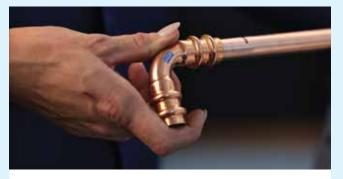
**7.** Insert the fitting, slightly rotating the fitting whilst sliding it onto the copper tube.
