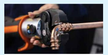
**11.** Place the jaw over both beads of the fitting at a right angle to the copper tube. Ensure the two beads of the fitting fit into the two corresponding grooves of the press jaw. Check the fitting is still fully engaged to the insertion depth mark and once the jaw and fitting is correctly engaged, initiate the pressing process by holding the start button.
