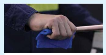
**4.** Clean and smooth the tube surface using an abrasive pad, emery paper or a soft medium grade scourer. Ensure the tube surface is free of indentation, scratches, deformation, oxidation and dirt or debris.
