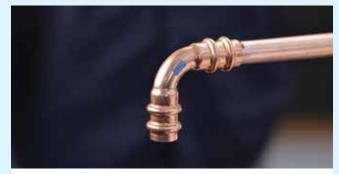
**8.** Slide the fitting all the way up to the insertion depth mark and until you make contact with the fittings stop. It is critical that full insertion depth has been achieved before pressing.
